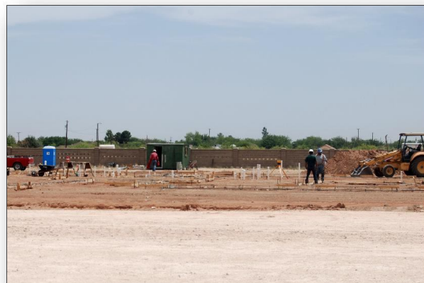
Construction progress May 2008
